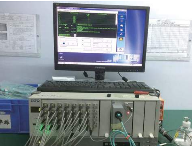
EXFO 32 port Multimode Insertion Loss & Return Loss
